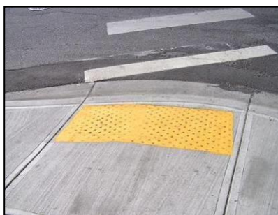
A curb ramp with truncated domes
