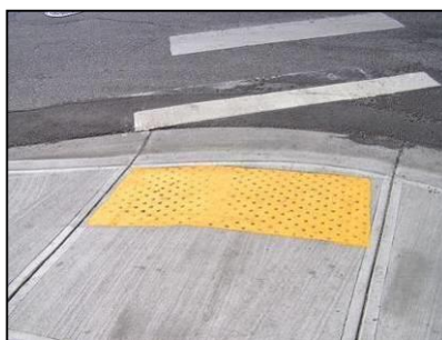
A curb ramp with truncated domes
